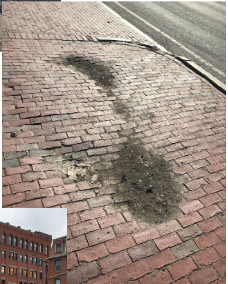
Photo of the poor state of repair on a sidewalk along Cambridge Street. The poor quality of the walkways create dangerous situations for pedestrians, especially those with mobility issues that frequently need to access MGH.
