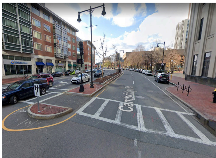
Sample cross-section of Cambridge Street at Sudbury Street. Buildings average 4-6 stories with some notable exceptions such as the high rise on the right side in the distance (Google Maps, 2022).
